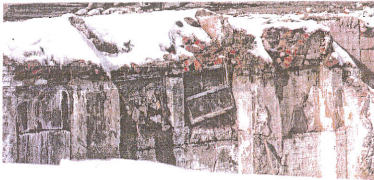
Dutchess County public works crews will begin filling the former Nelson House Hotel Annex basement with gravel next week. DARRYL BAUTISTA/POUGHKEEPSIE JOURNAL
